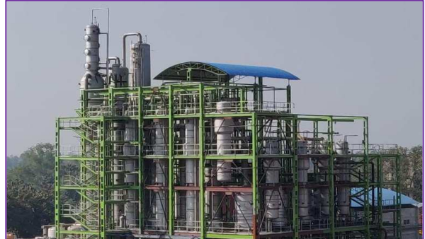
Solvent Recovery Plant
