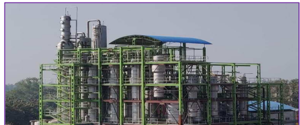
Solvent Recovery Plant
