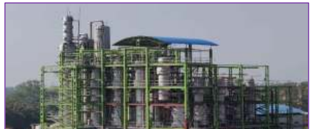
Solvent Recovery Plant
