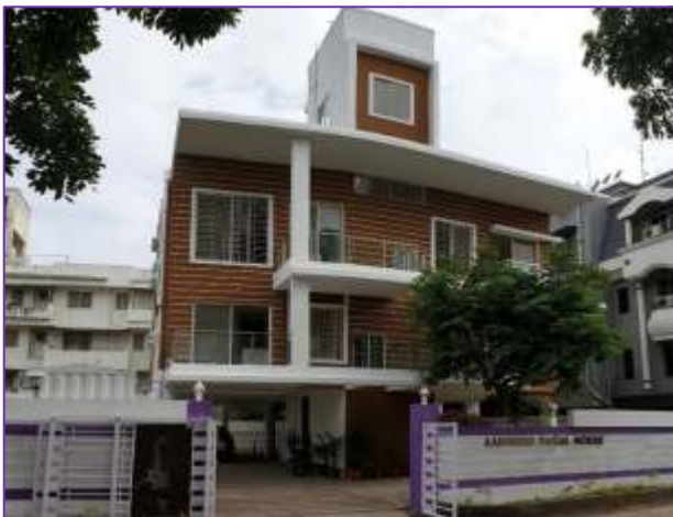
EXCEL – PUNE HEAD OFFICE
