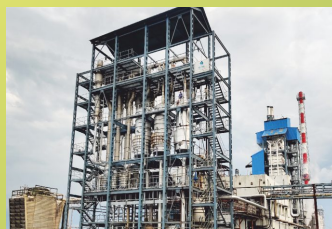
EID Parry (Andhra Pradesh) Evaporation Plant
