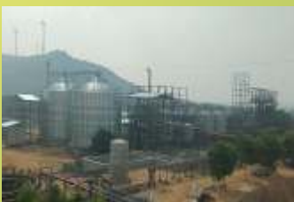
RJC Agro Ltd., Andhra Pradesh Grain Distillery
