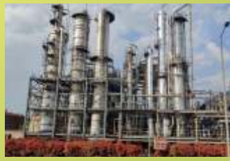
Hermes Distillery Ltd Karnataka Grain ENA with DDGS Plant
