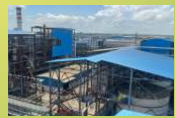
India Glycols Limited, Uttar Pradesh - Grain Distillery
