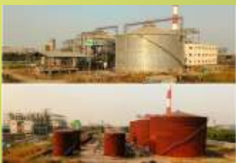
KRIBHCO Green Energy, Gujarat Grain Distillery
