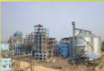
Ambashakti Bioenergy Pvt. Ltd., Madhya Pradesh - Grain Distillery
