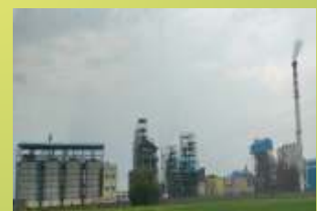
Ethane Bio-fuel Pvt. Ltd., Rajasthan - Grain Distillery
