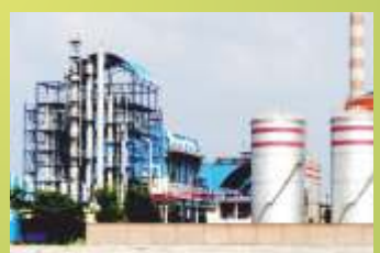
YAPL (Maharashtra) - Molasses ENA / Ethanol Distillery With BMSW / RW Evaporator
