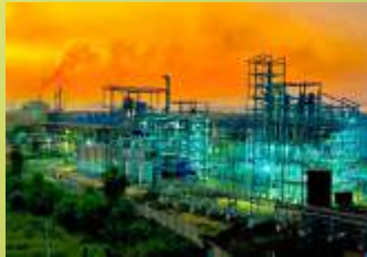
UKR Industries Ltd., Madhya Pradesh – Grain Distillery
